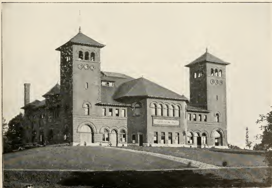
AUDITORIUM HALL. Main building of the Northfield Schools
